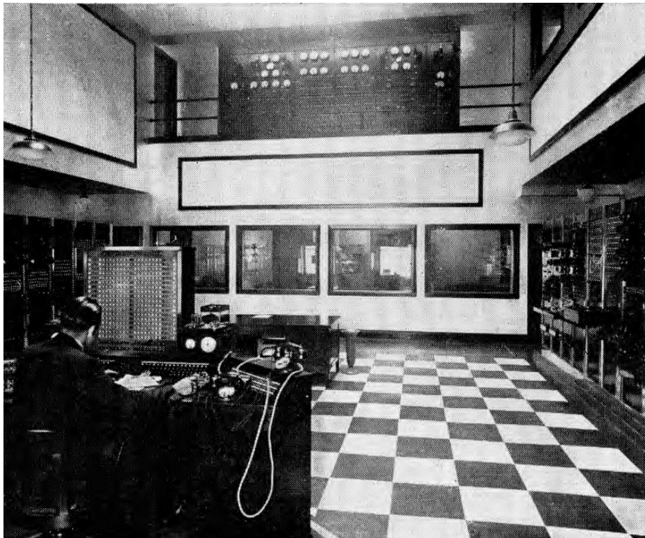
[Above left] Merchandise Mart NBC Master Control showing full wall of patch panels at left.
