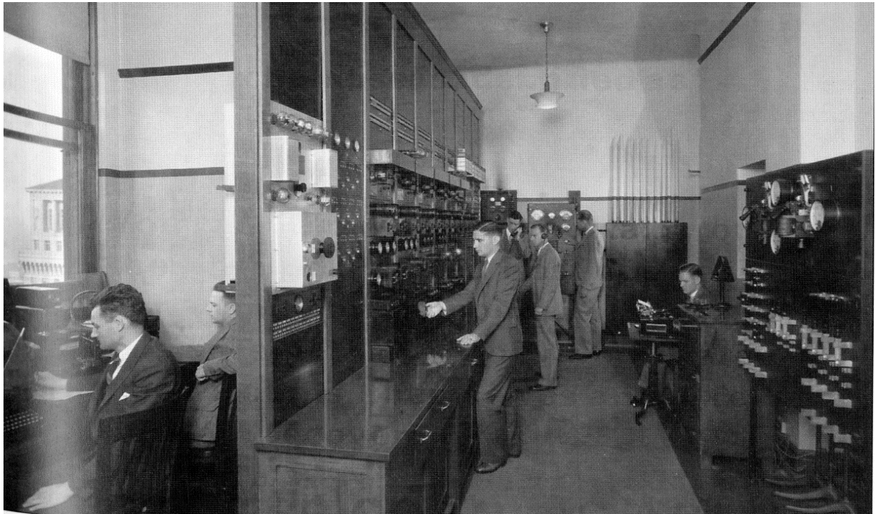
(Below) Main transmission room through which all network feeds were controlled [Courtesy of John Schneider]
