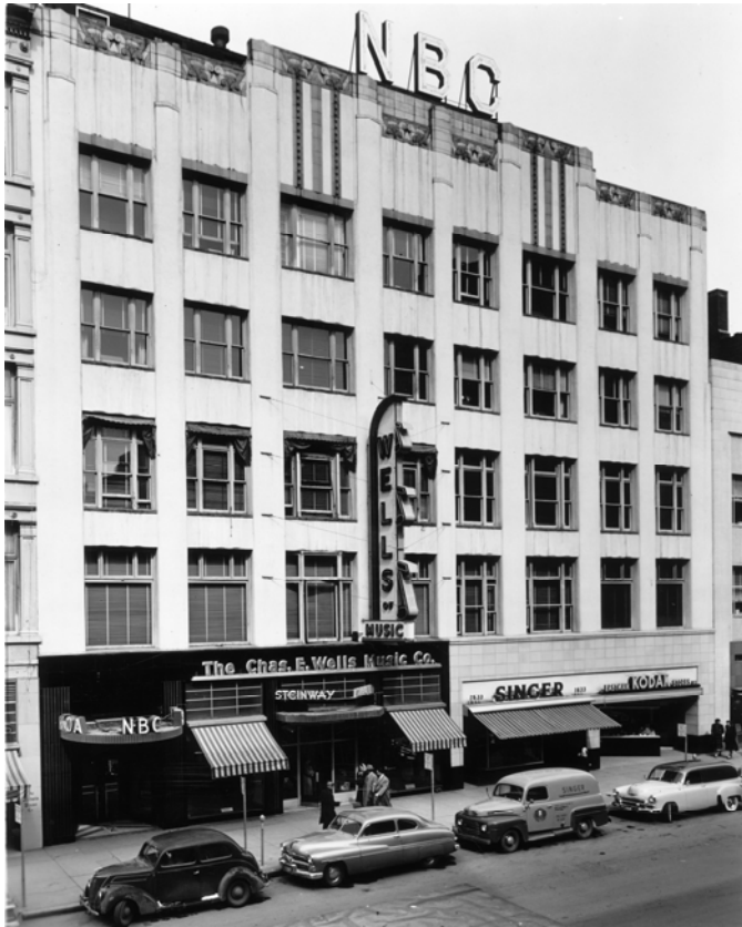
[Left] Radio City Denver (also later known as the Wells Music Building) exterior
