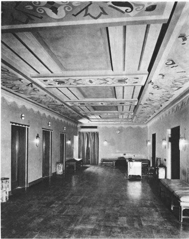
Corridor with elevators
