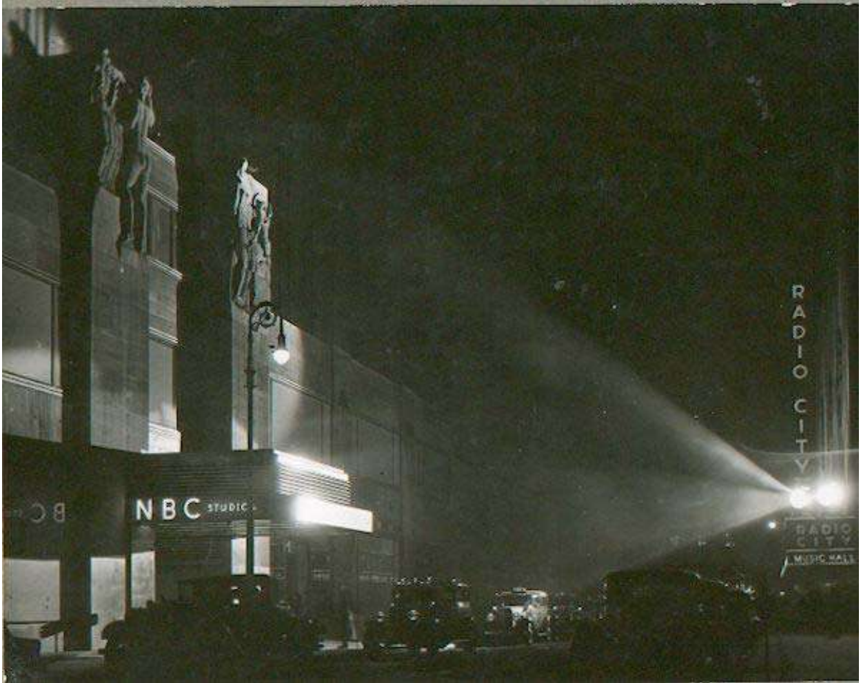
(Above) NBC main entrance at night [NBC/NBCU NUP_141759_0001.jpg]
