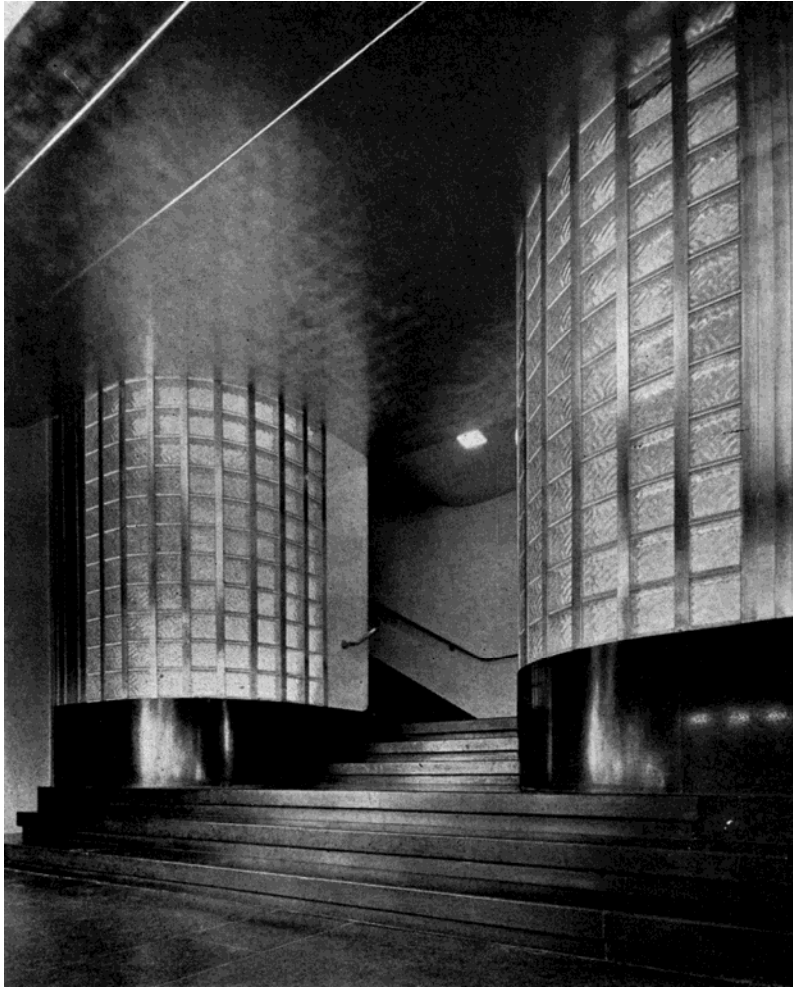
(above) Staircase at main lobby rear .
